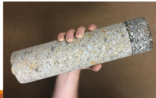
Sample from a Full Depth Reclamation (FDR) repair
